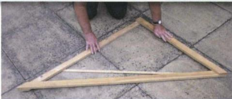
A large setsquare for setting out
